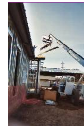
The roof going on!
